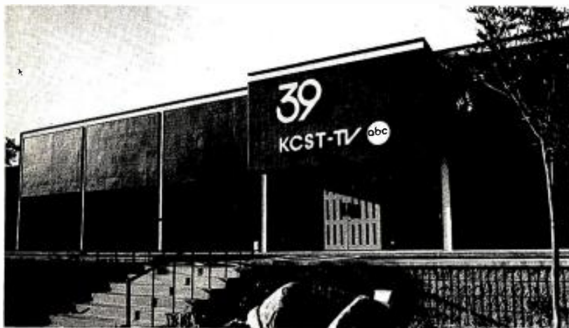
New home. KCST-TV. Storer Broadcasting Co.'s San Diego UHF station now operates out of a newly-completed 30,000-square-foot broadcast center. At reconstruction and remodeling costs of more than $850,000, Storer added an additional 8,000 square feet and revamped the entire interior of the building which once had been used as a ballpoint pen factory. KCST-TV is an ABC affiliate.
